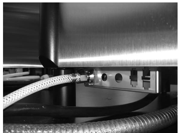
INSTALL WATER SUPPLY LINE
